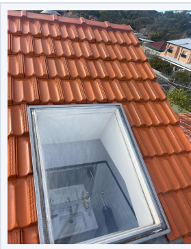
13 Skylight reset & sealed Flashed into a restored roof
