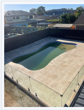
10 Travertine pool surround Coping and paving laid
