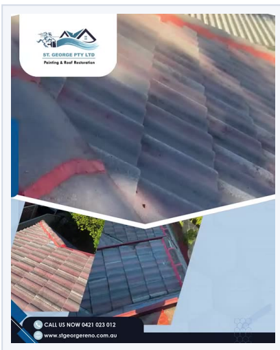
FIG. 14 Full roof restoration. Job footage, 58 seconds.
