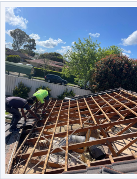
09 Full strip & re-batten Taken back to frame and rebuilt
