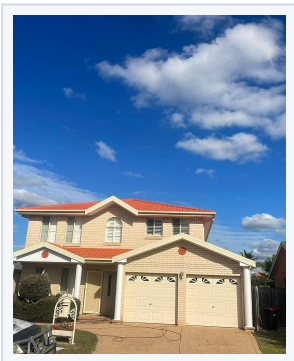
04 Completed roof restoration Full clean, re-bed, re-point and coating
