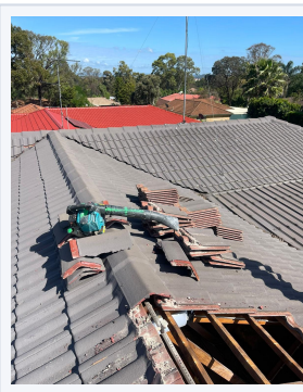
06 Re-bedding & re-pointing Ridge capping stripped and re-bedded
